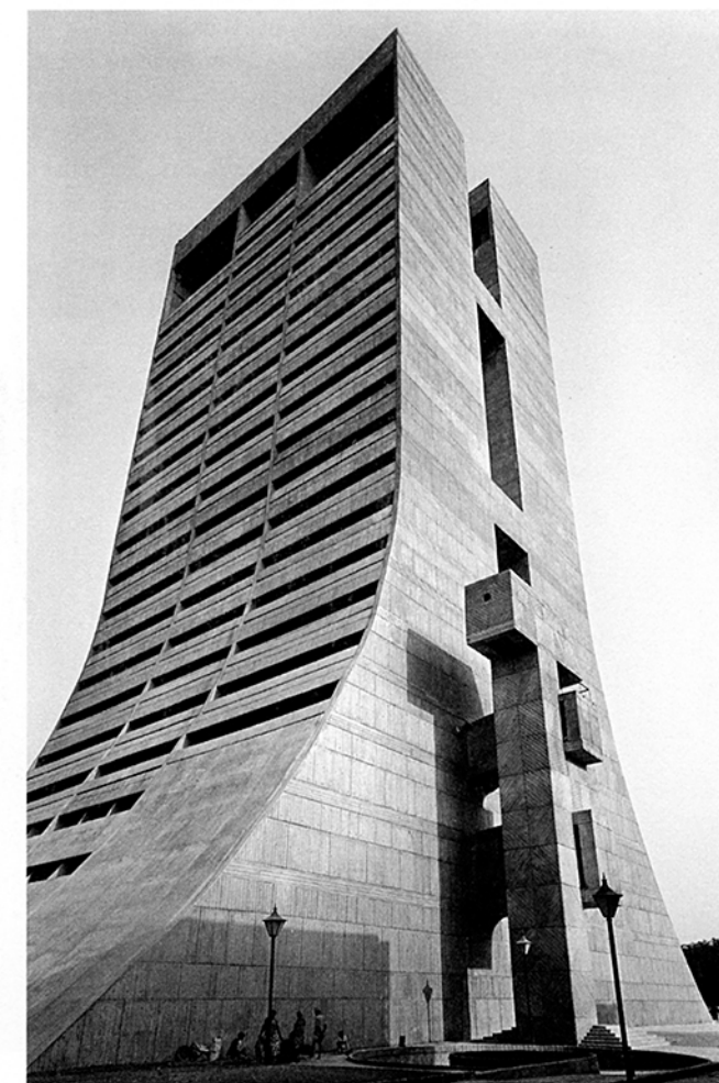
New Delhi Municipal Council building, Palika Center, 1983, Courtesy: Madan Mahatta/Photoink.
