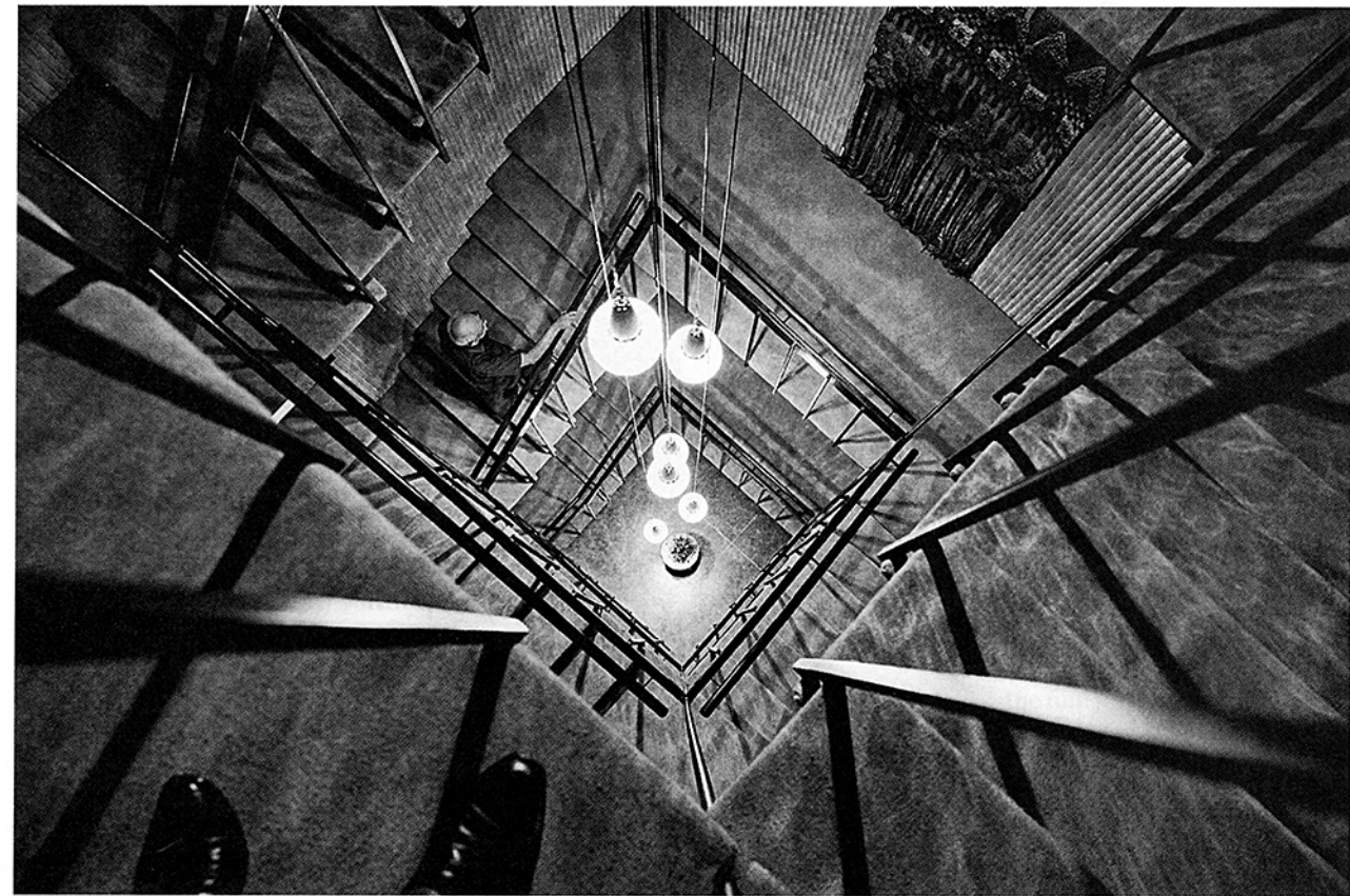
Joseph Allen Stein walking up the staircase, Ford Foundation office, 1968. Architect: Joseph Allen Stein. Photo Courtesy Madan Mahatta/Photoink
