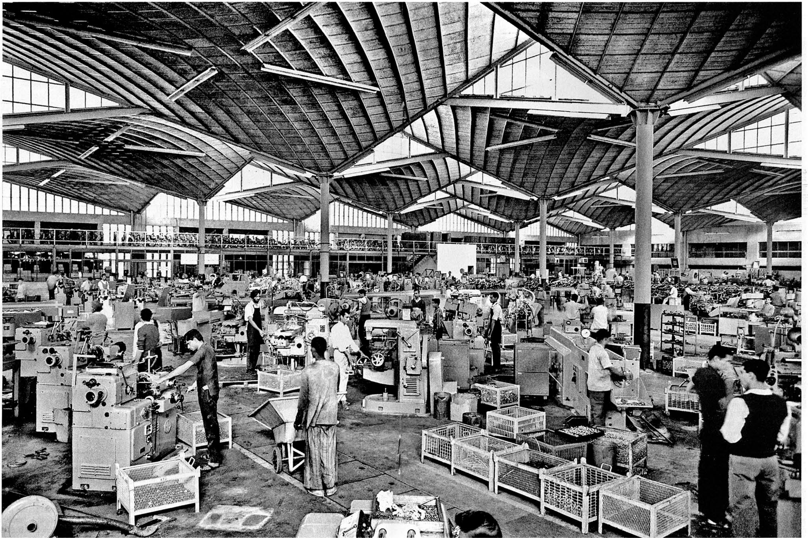
INSIDE THE ESCORTS factory, I, 1964. Architect: Joseph Allen Stein. Mahatta's depiction of the Escorts factory demonstrates how the design of the building facilitates the assembly line of production.
